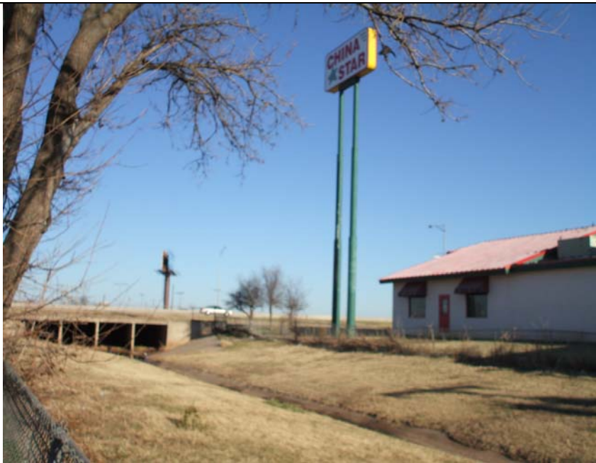
Photograph depicts the Plum Creek Drainage Ditch and China Star Restaurant located south of the Subject Property.
