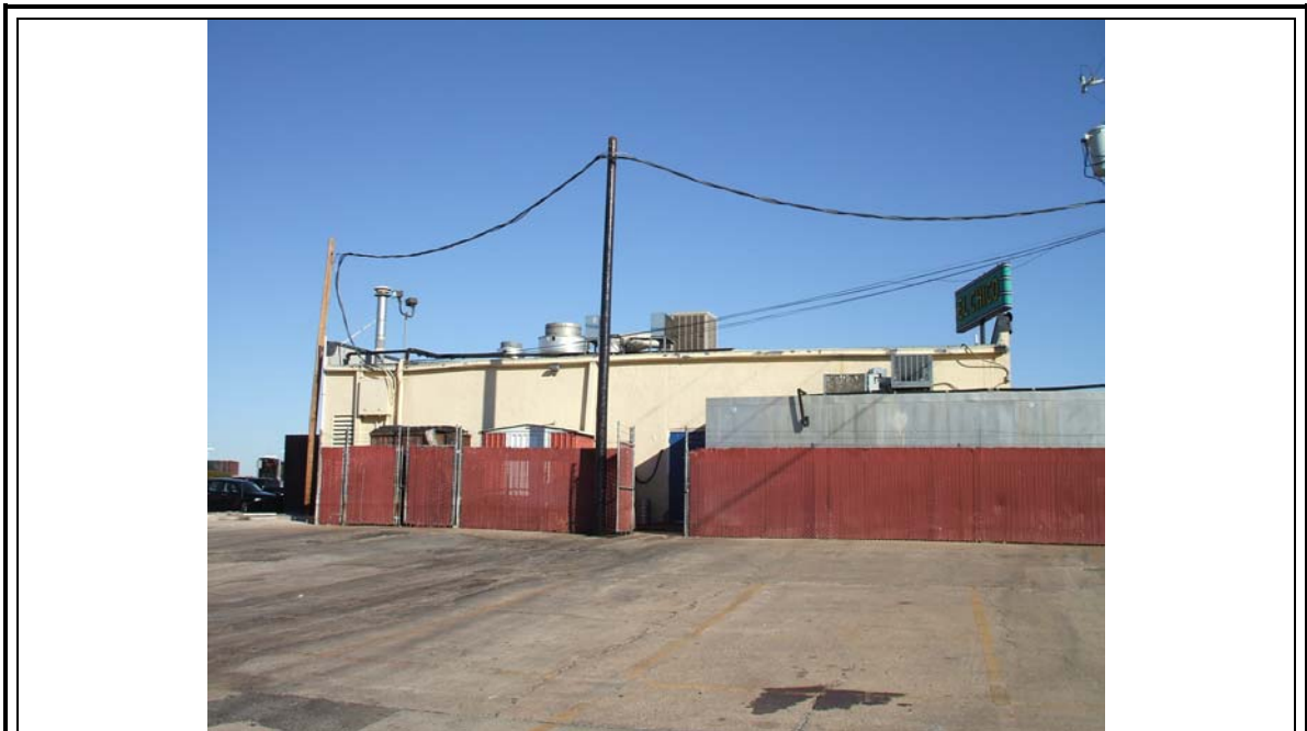
Photograph depicts the west side of the building, view facing east.
