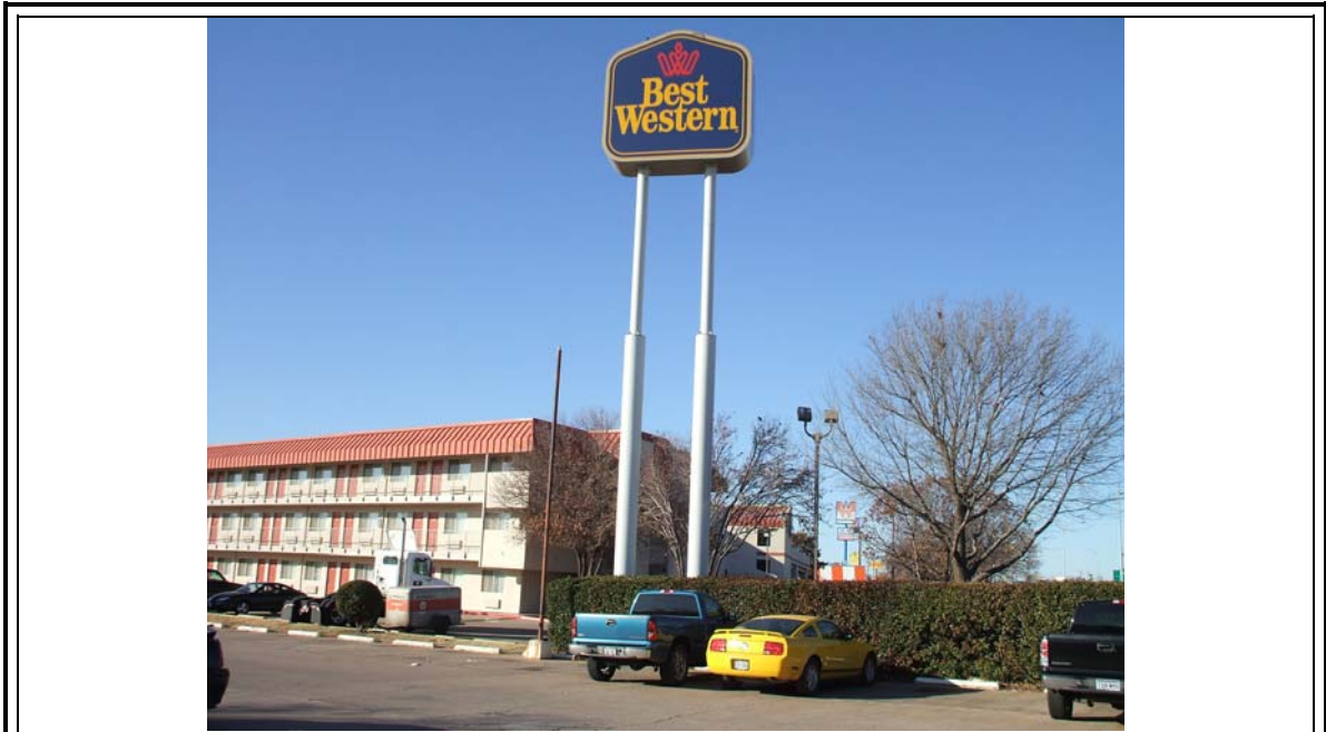
Photograph depicts the Best Western located north of the Subject Property.
