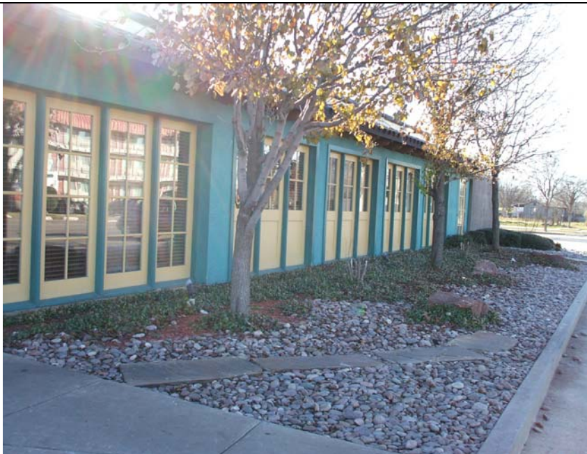
Photograph depicts the north side of the building, view facing southwest. This is the former patio that was enclosed in 1993.
