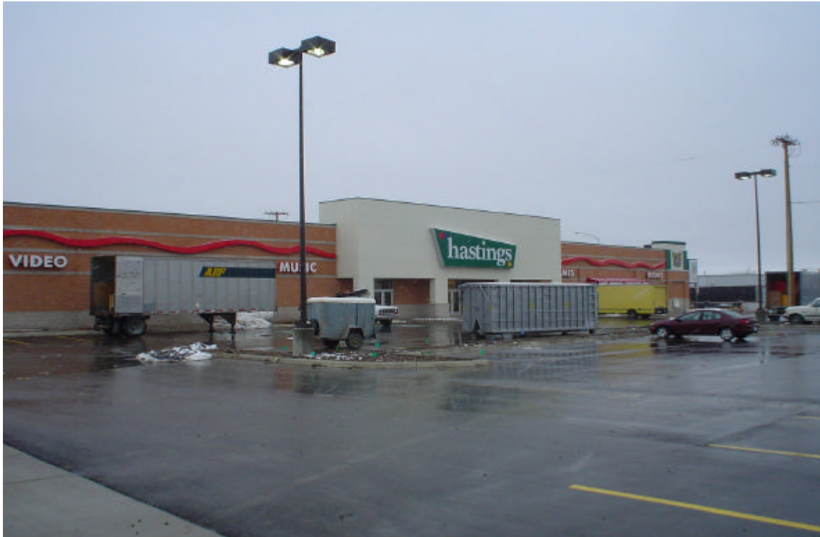
Exterior - Viewing Northwest
