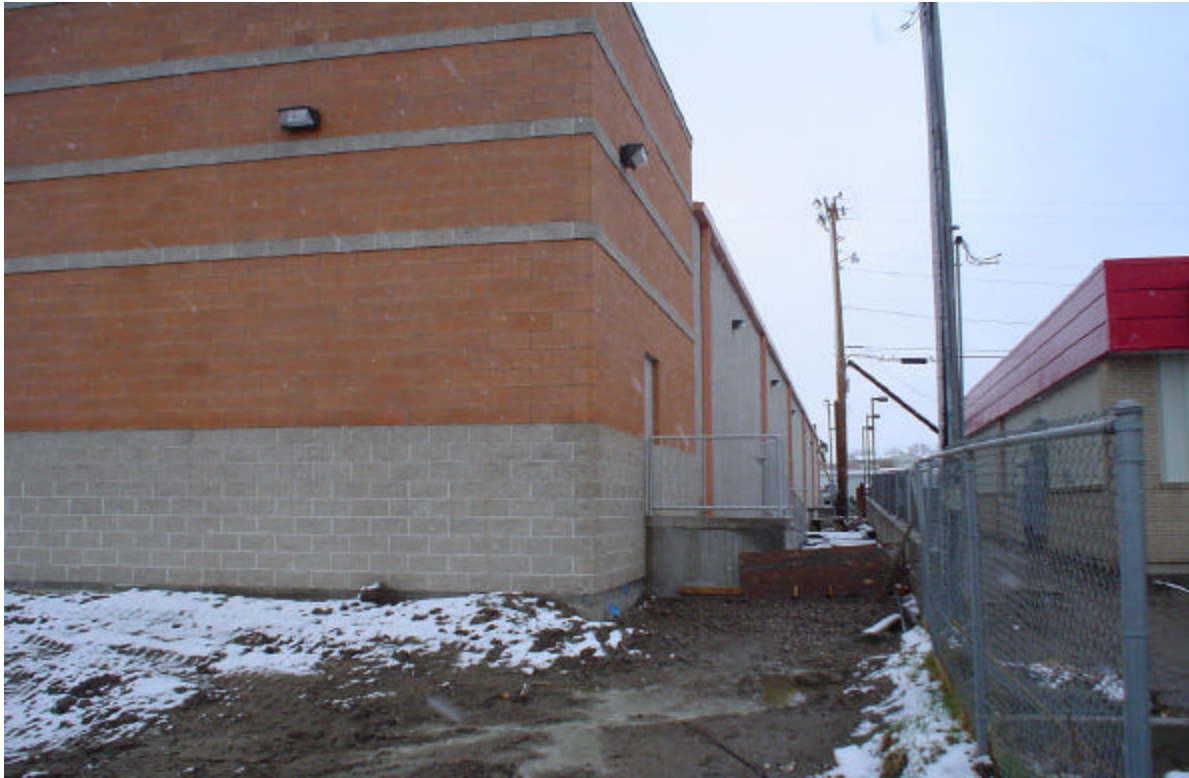
Exterior - Viewing Southeast
