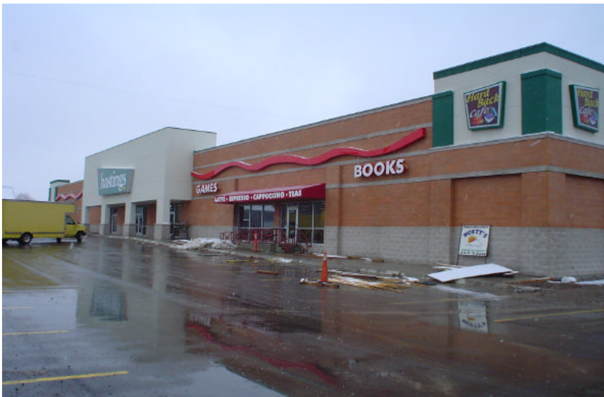
Exterior - Viewing Southwest
