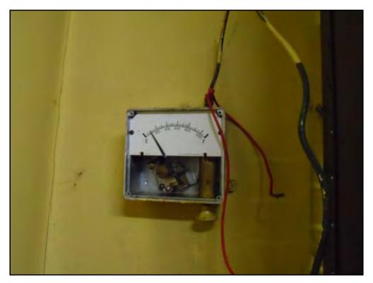
21 : A view of the former UST tank product gauge fixed to the north interior wall in the basement in the general storage area, looking north. The gauge is completely disconnected and is not currently in use.
