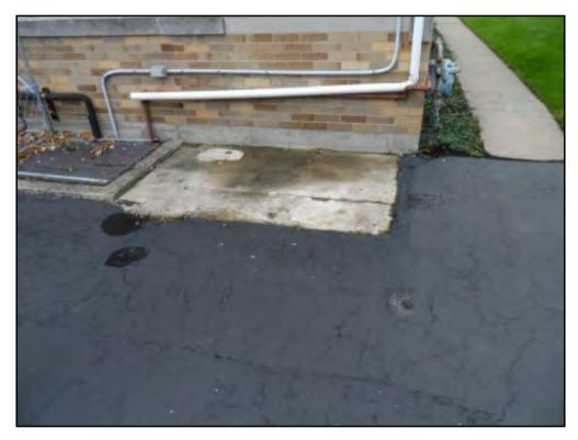
9: A view of a stained concrete pad on the north exterior wall, at the northwest corner of the Site Building. This general area is the approximate location of the former UST locations, and evidence of an old chainlink fence is visible in the concrete and asphalt (post holes for the fence). The grate immediately left of the concrete pad is open to the basement boiler room.
