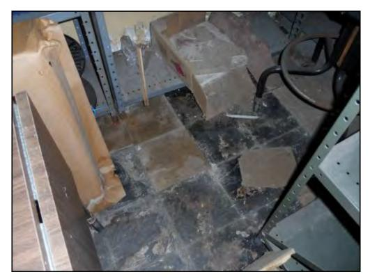
22 : A view of 9-inch by 9-inch floor tiles and floor mastic. (suspected to be PACM) in the general storage area in the basement.
