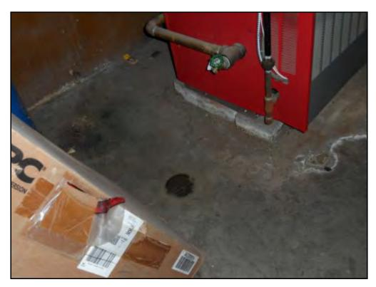
16 : A floor drain was observed south and adjacent to the boiler. The current status of the drains and where it discharges to was not reported.
