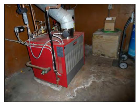
15 : A view of the basement boiler room, including a view of the former air sparge motor and pump box, water heater tank, and associated equipment. De minimis staining is shown at the foot of the boiler.
