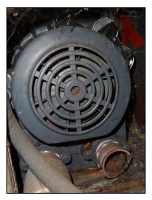
17: The air sparge motor was observed inside a wooden box next to the boiler. The motor was completely disconnected, and has not been used since the closure of the NYSDEC spill report.
