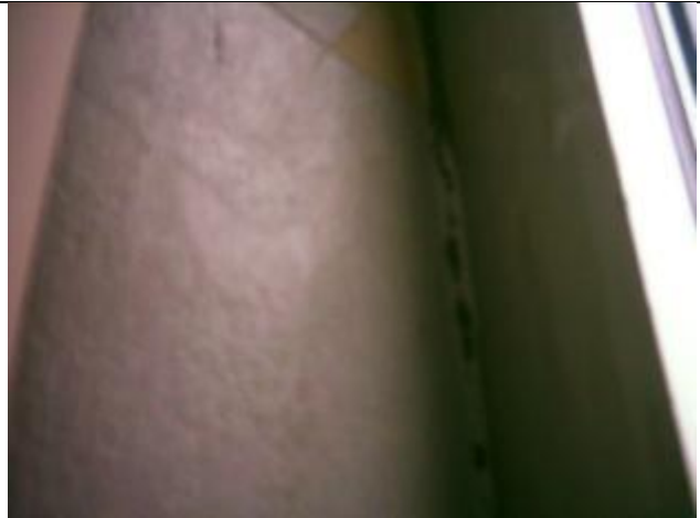
HA-3,4: Wall Plaster (White & Brown Coat)
