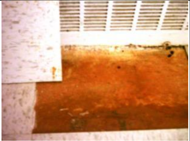
HA-20, 21: 12x12 Floor Tile and Mastic
