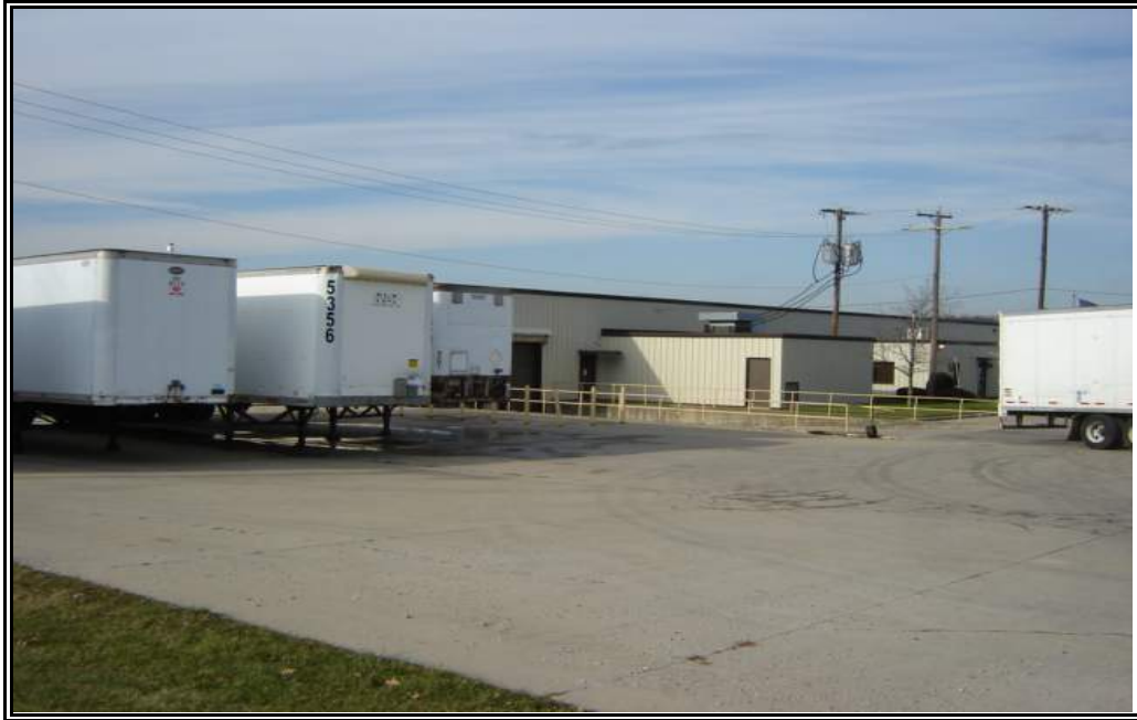
View of the Plant #2, looking northwest from the southeast corner of the site.
