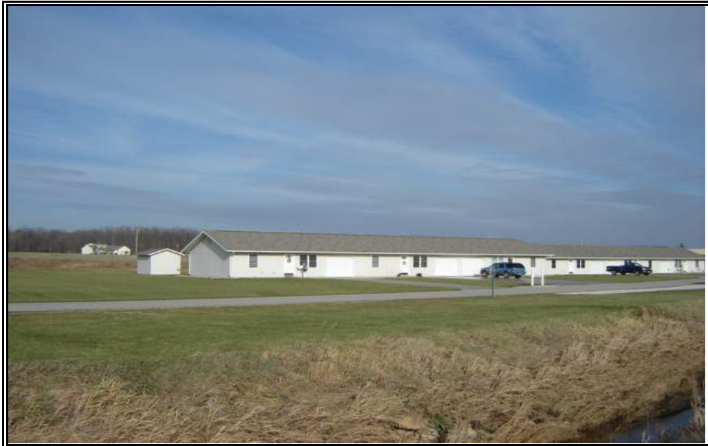
View of the adjacent property to the north of Plant #2.
