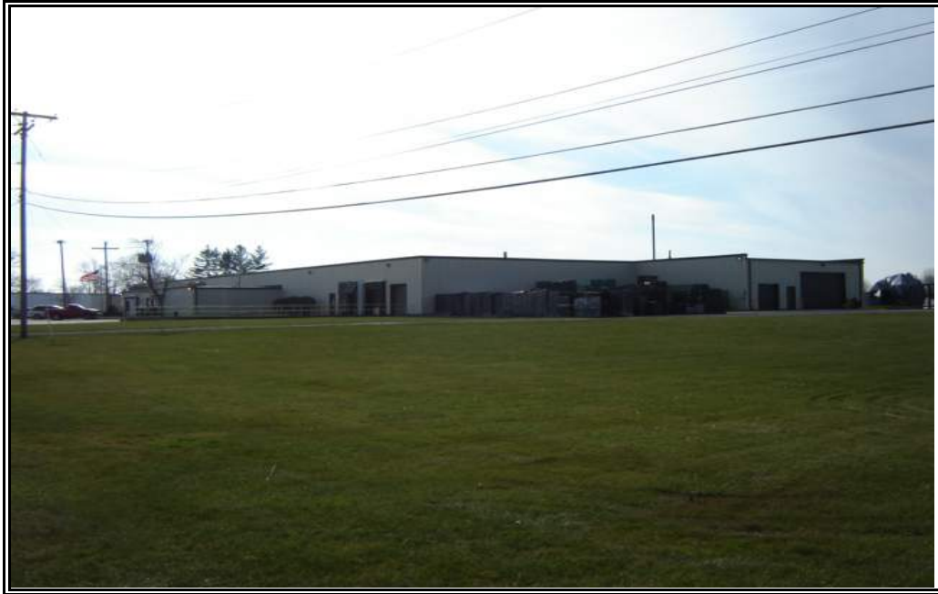
View of Plant #2, looking southwest from the northeast corner of the site.
