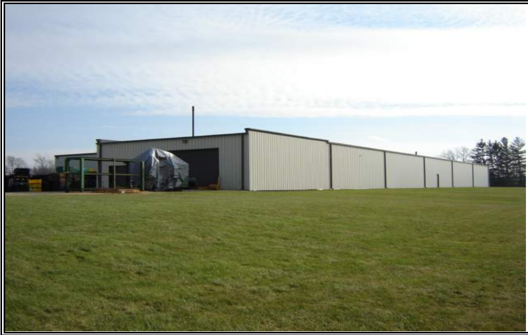
View of the subject property (Plant #2), looking southeast from the northwest corner of the site.
