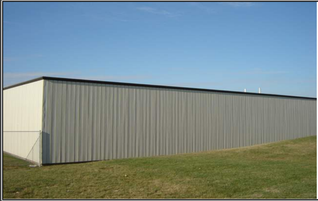
View of the subject property (Plant #1), looking northwest from the southeast corner of the site.
