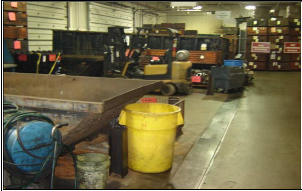
View of the chip dumpsters and trench drain system in the oil/chip room in Plant #1.
