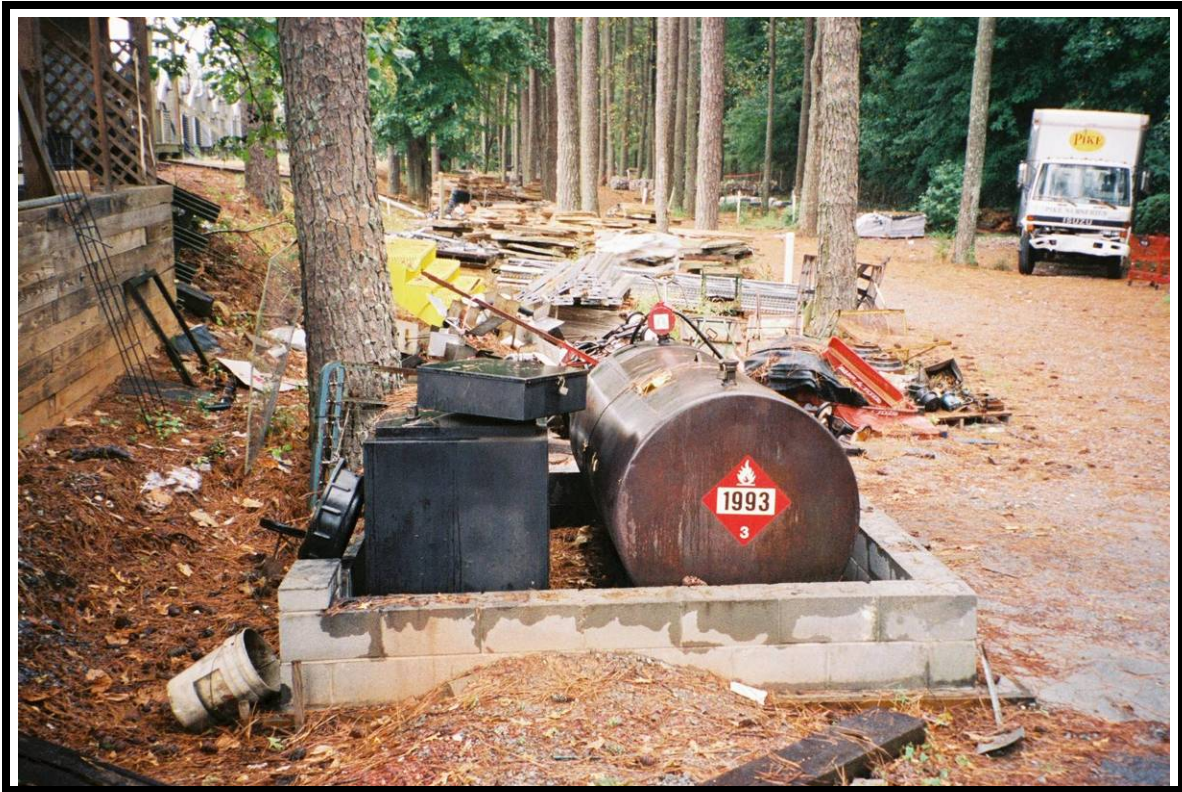
3. View of the ASTs to the southwest corner of the interior wholesale / rocks and aquatic building.
