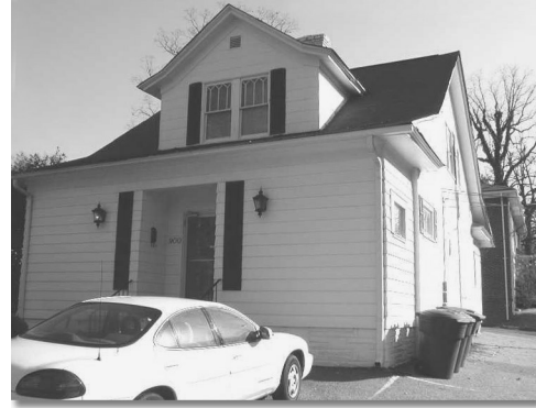
The inappropriate enclosure of the front porch of this residential structure for commercial use, prior to historic district designation, compromised the integrity of this historic structure.
