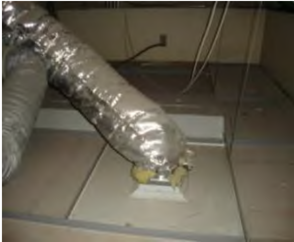
HA-26: Fiberglass Duct Insulation
