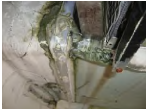
HA-21: HVAC Caulk
