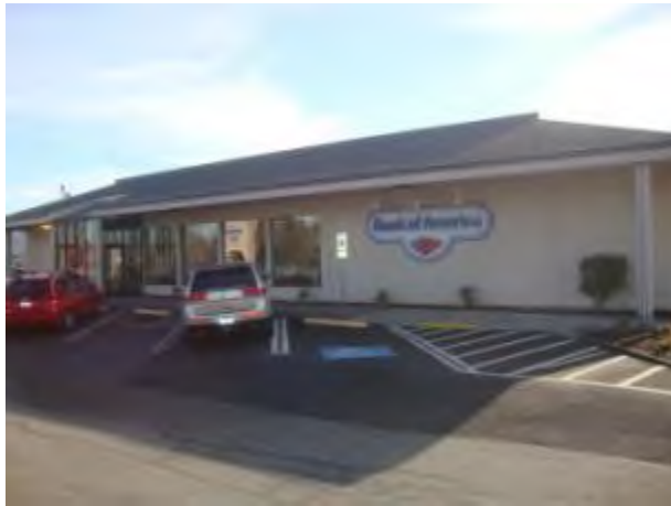
Front View of the Building
