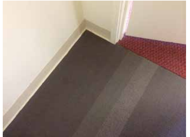
HA-31: Brown Carpet; HA-32: Clear Carpet Adhesive; HA-33: Residual Brown Mastic
