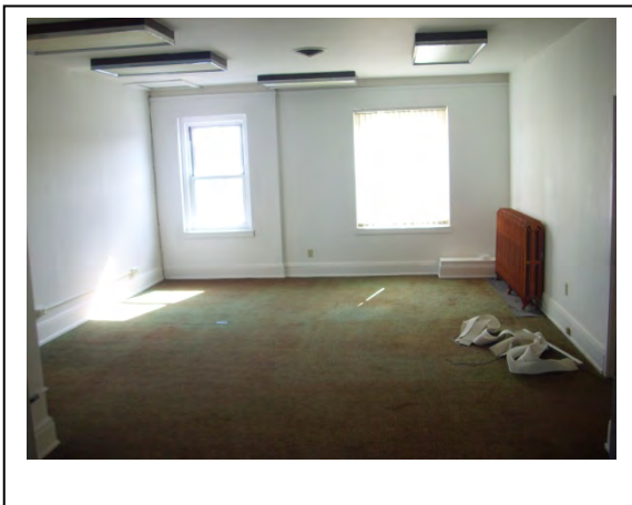
HA - 21: 2'x4' Fissured ceiling tiles.
