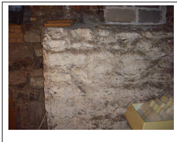
HA - 4: Surface plaster.
