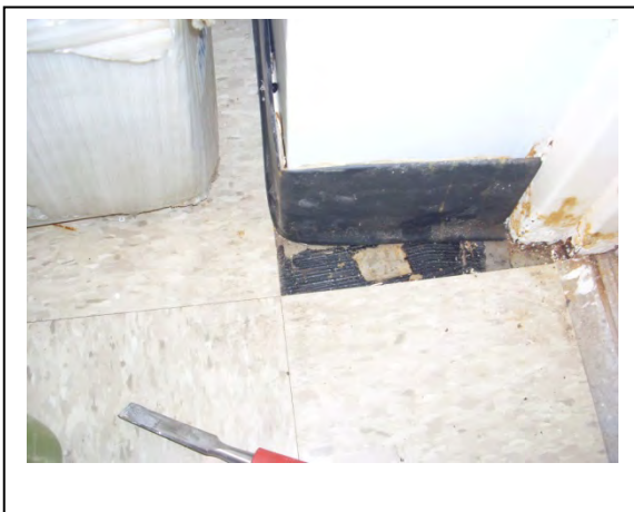
HA - 11/12: 12" x12" Gray marbled floor tile; Mastic for Gray floor tile.
