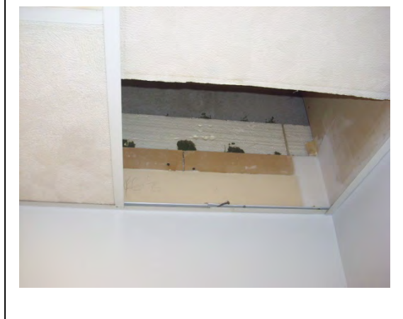
HA - 25/26: Joint compound and drywall.
