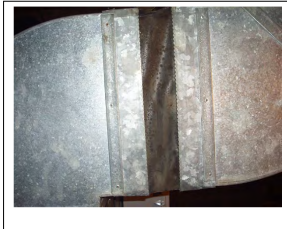
HA - 28: HVAC flex connector.
