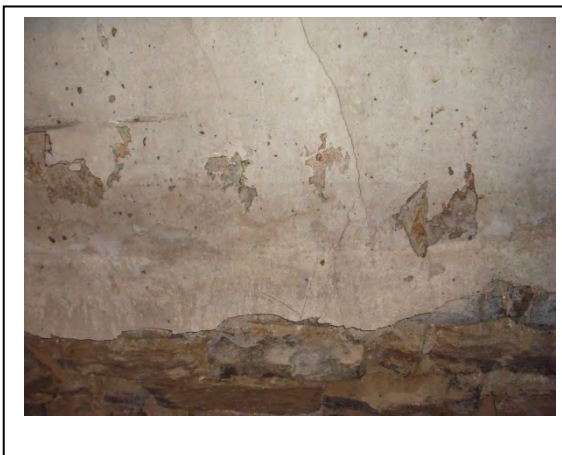
HA - 3/6: Plaster skim coat and stone grout.
