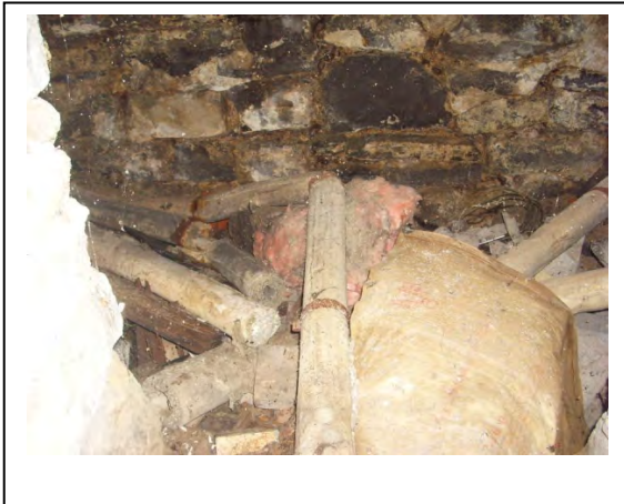
HA - 1: Air cell in crawl space.
