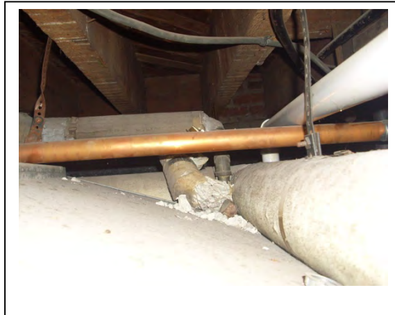
HA - 2: Severely damaged muddied fitting.
