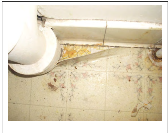
HA - 22/23: Vinyl floor sheet and associated adhesive.
