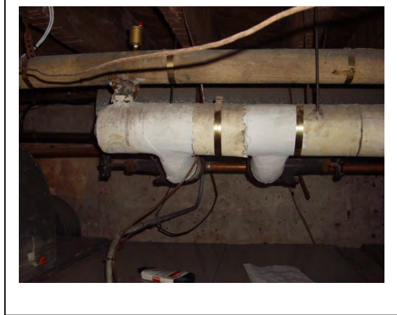
HA - 1/2: Aircell pipe insulation and muddied fittings.
