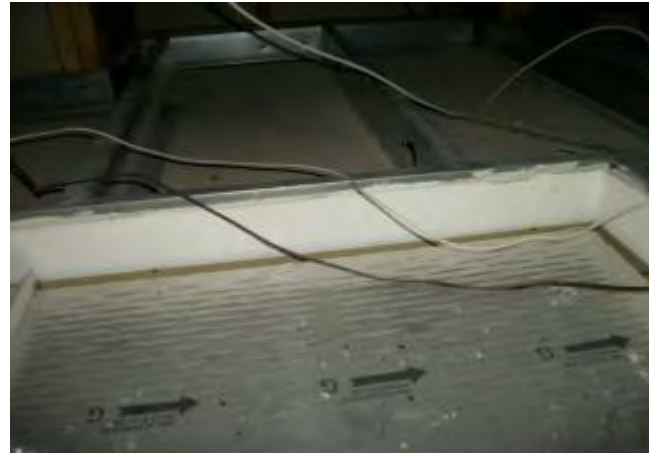
HA-1: White Gypsum Board, HA-2: Associated White Joint Compound
