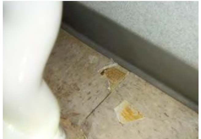
HA-15: Gray Vinyl Sheet Flooring (2 nd layer), HA-16: Associated Yellow Floor Tile Mastic, HA-17: Gray Vinyl Sheet Flooring (3 rd layer), HA-18: Associated Yellow Floor Tile Mastic
