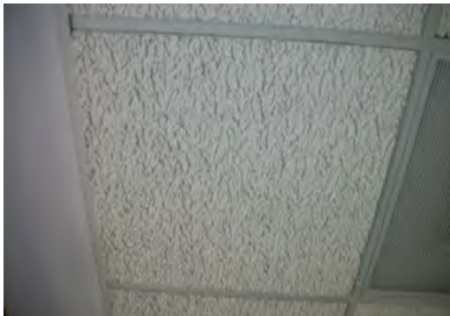
HA-3: White 2' x 2' Suspended Ceiling Tiles
