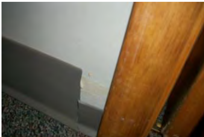
HA-5: Gray 4" Vinyl Cove Base, HA-6: Associated Yellow Cove Base Mastic
