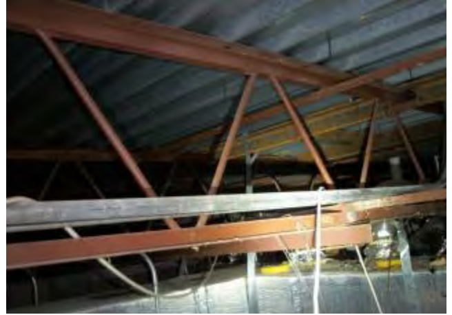
HA-12: Yellow Fiberglass HVAC Duct Insulation
