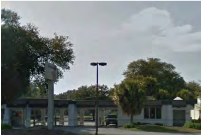
View of the Front of the Building
