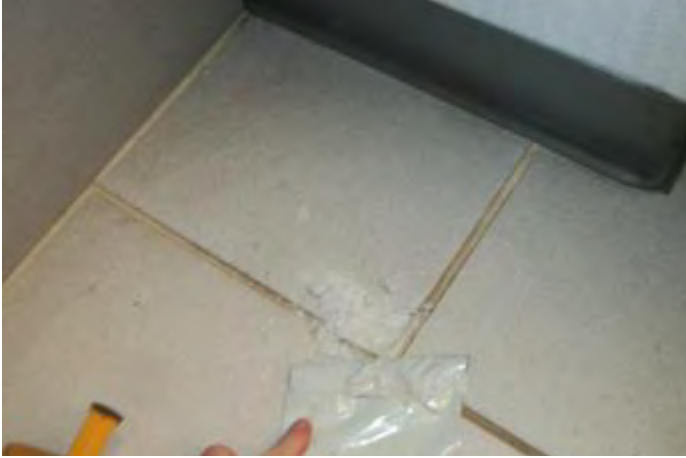
HA-9: Gray 12" x 12" Ceramic Floor Tile, HA-10: Associated Gray Floor Tile Grout, HA-11: Associated Gray Floor Tile Adhesive
