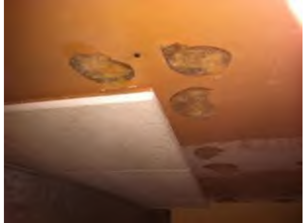
HA-19: 1' x 1' Ceiling tiles - Glue On HA-33: Brown ceiling tile glue
