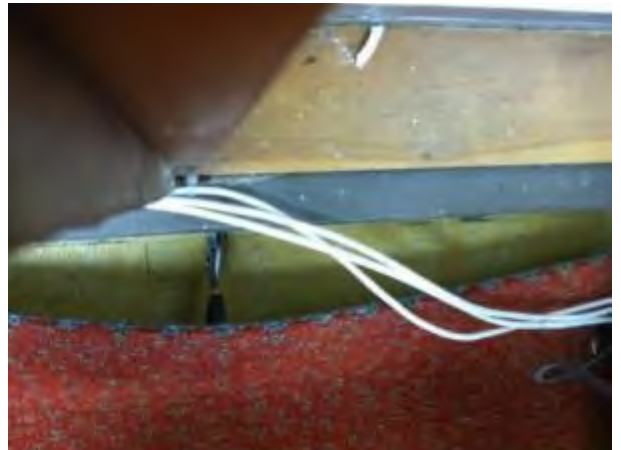
HA-24: Brown & white specks floor tiles (Under Carpet) HA-25: Black floor tile mastic
