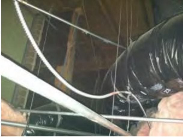
HA-50: Pink fiberglass batt insulation HA-51: Black plastic-wrapped fiberglass duct insulation
