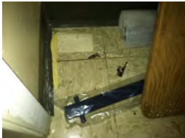
HA-45: Beige sheet flooring (beneath vinyl floor tiles) HA-46: Brown sheet floor backing
