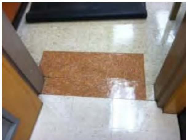
HA-12: 12" x 12" Tan with brown streaks floor tiles HA-13: Black floor tile mastic
