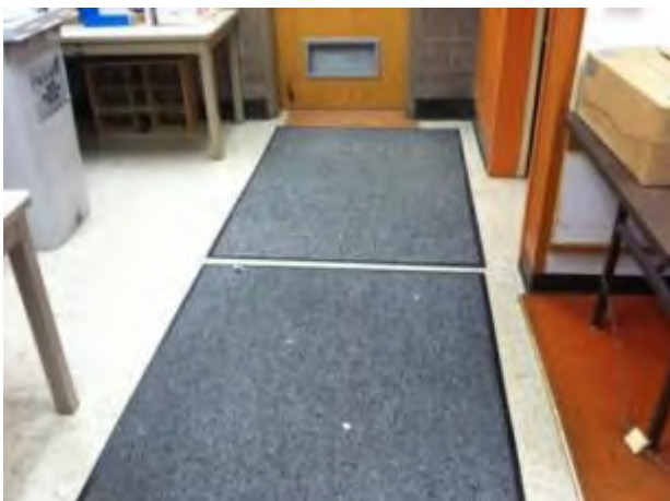
HA-27: 12" x 12" Beige with large brown streaks floor tiles HA-28: Black floor tile mastic HA-29: White levalastic beneath HA-27/HA-28
