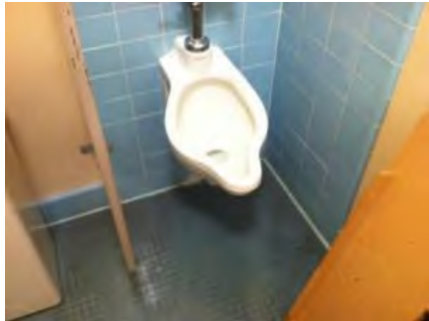
HA-39: Blue 4" x 6" ceramic wall tiles/cove base HA-40: Tile adhesive HA-41: White tile grout
