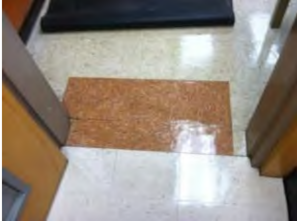
HA-17: 12" x 12" White with tan streaks floor tiles HA-18: Black floor tile mastic
