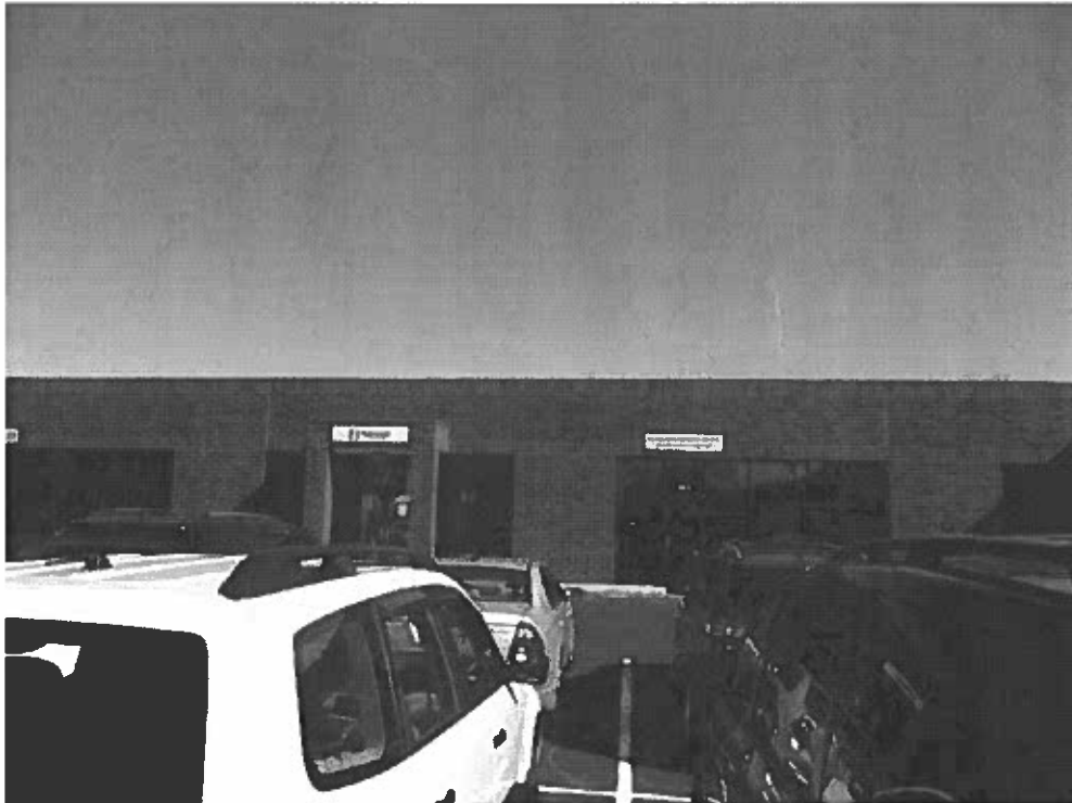
Photo #6: View of the western boundary of the Site. Airport Avenue and pad-mounted transformers can be seen.
