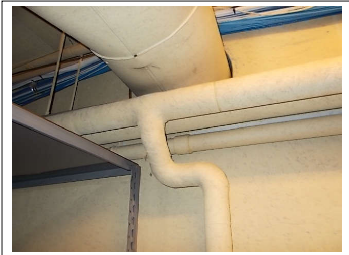
View Of: Pipe fitting insulation, ACM (Sample 13)
