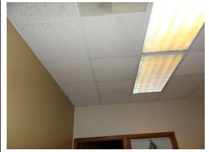
View Of: 2' x 2' ceiling tile, rough, recessed edges, non-ACM (Sample 3)
