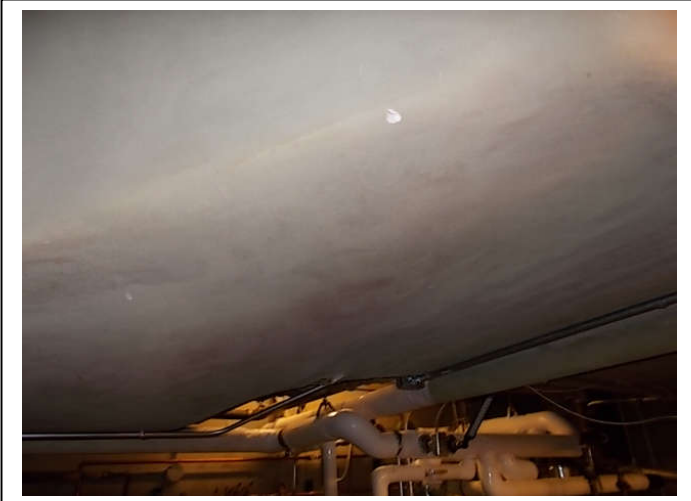
View Of: Boiler room plaster ceiling, non-ACM (Sample 9)
