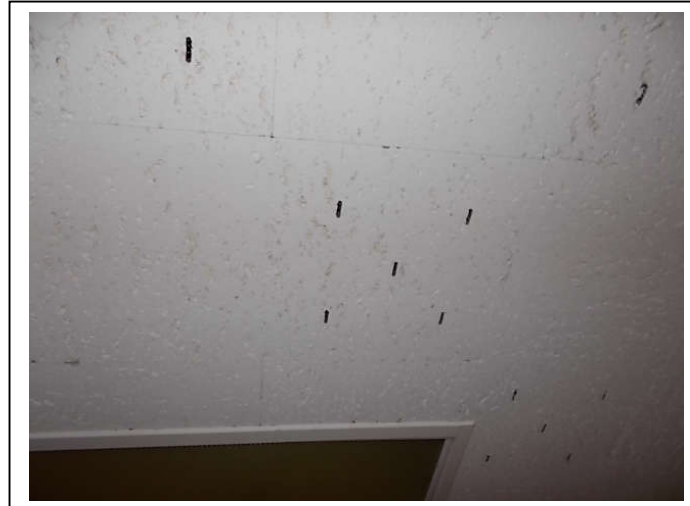
View Of: 1' x 1' concealed spline ceiling time, non-ACM (Samples 1, 10)
