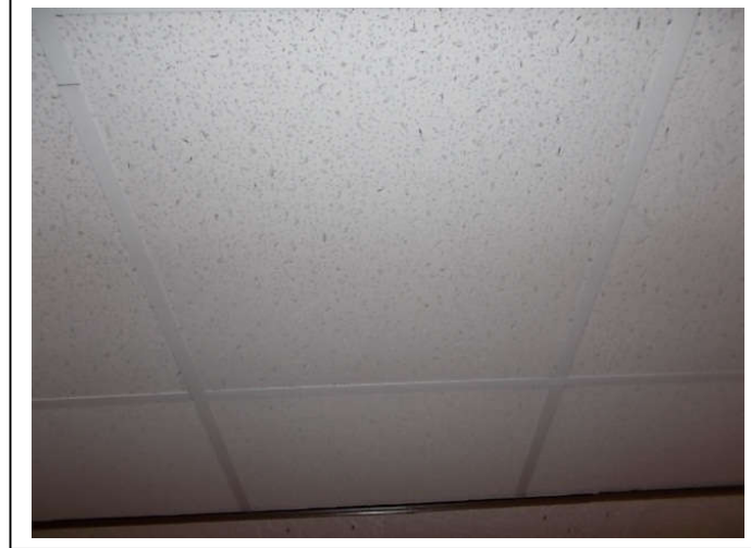
View Of: 2' x 2' Ceiling tiles, non-ACM (Sample 11)
