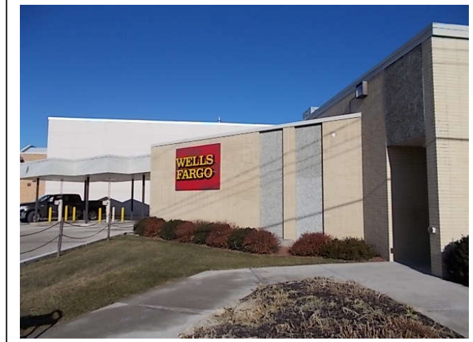
View Of: West side of building
