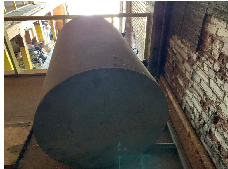
Representative Miscellaneous Storage of Items in Warehouse Basement
