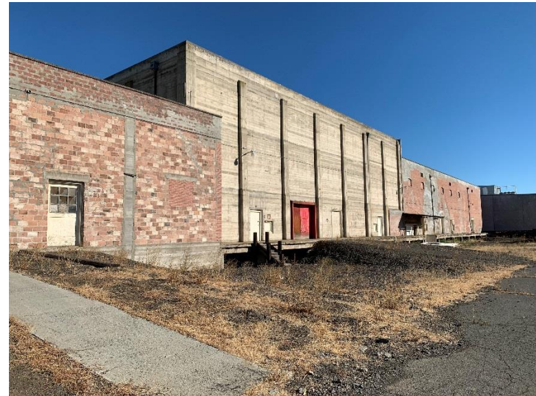
West Side of Warehouse – View to South
