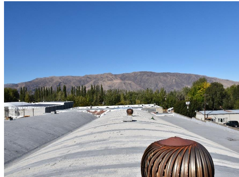
View of Northern Portion of Warehouse Roof – View to North
