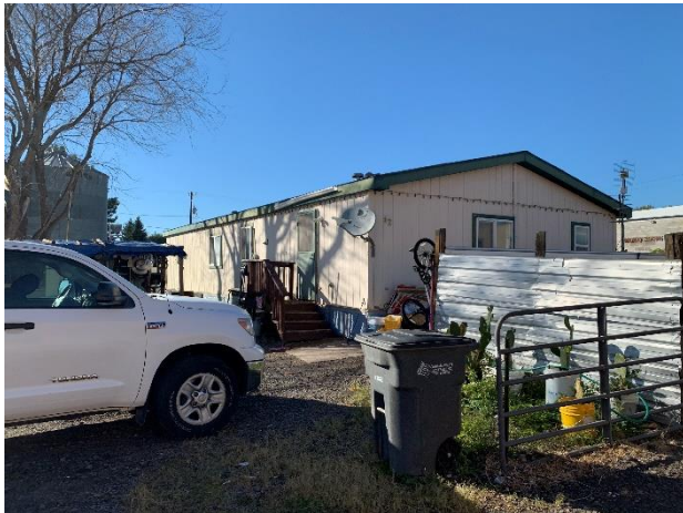
Mobile Home Unit in Northwest Portion of Subject Site
