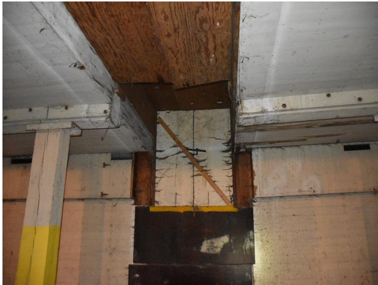
Representative Access Area Between Floors and to Building Exterior
