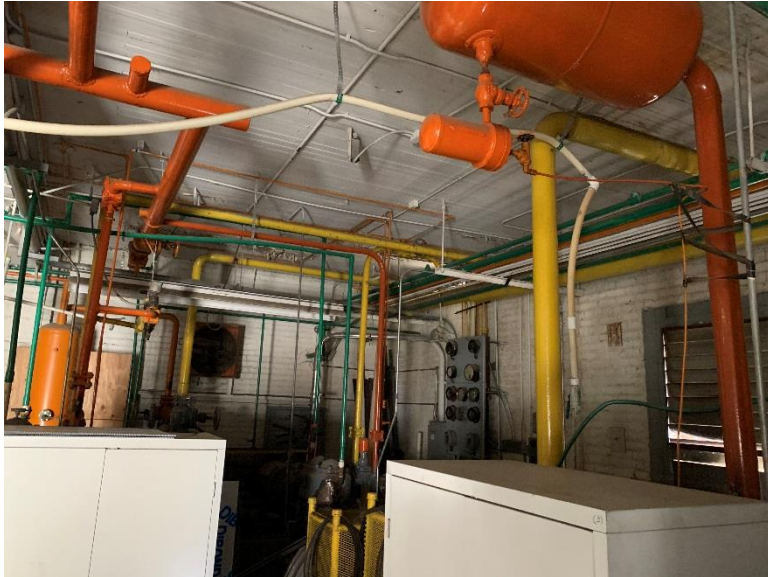
Interior of Western Portion of Mechanical Building
