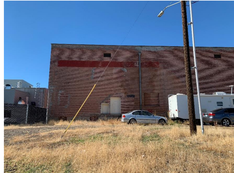
View of Warehouse and RV Parked in Southeastern Portion of Subject Site
