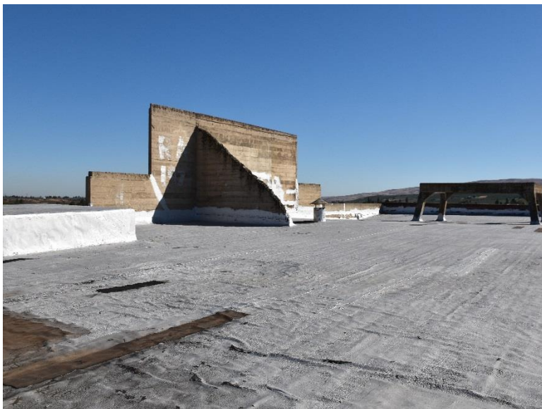
View of Central Portion of Warehouse Roof – View to Southeast
