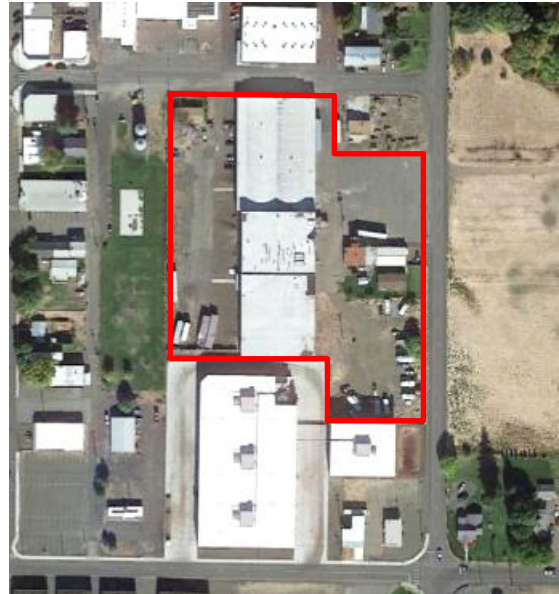
Subject Site Location
