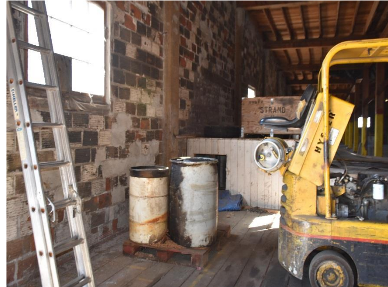
Forklift and Drums Stored within Northern Portion of Warehouse, Main Floor – View to South
