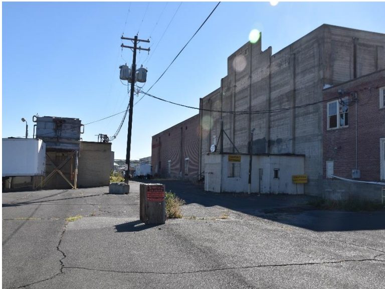
Exterior Portion of Warehouse, Eastern Exterior Wall – View to South
