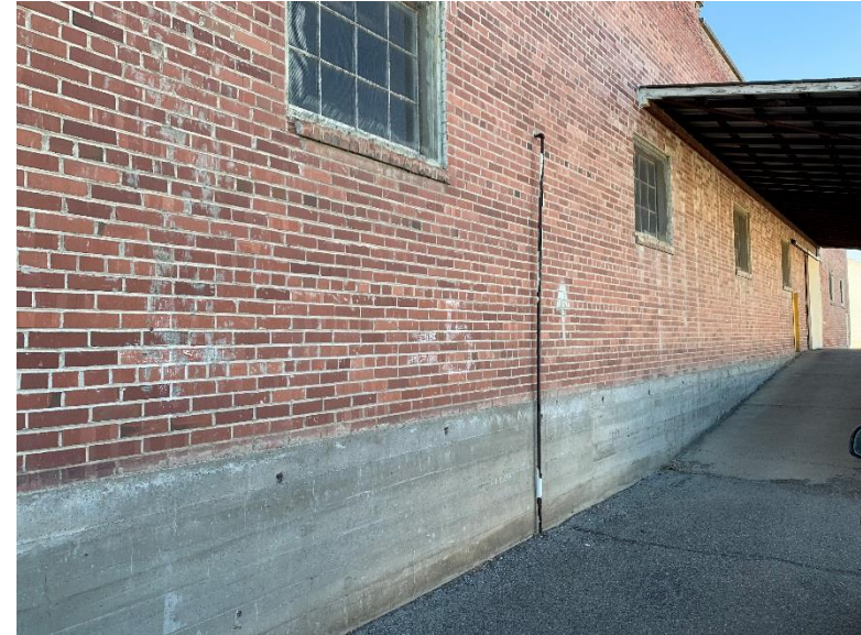
Northern Exterior Portion of Warehouse, Eastern Exterior Wall – View to North
