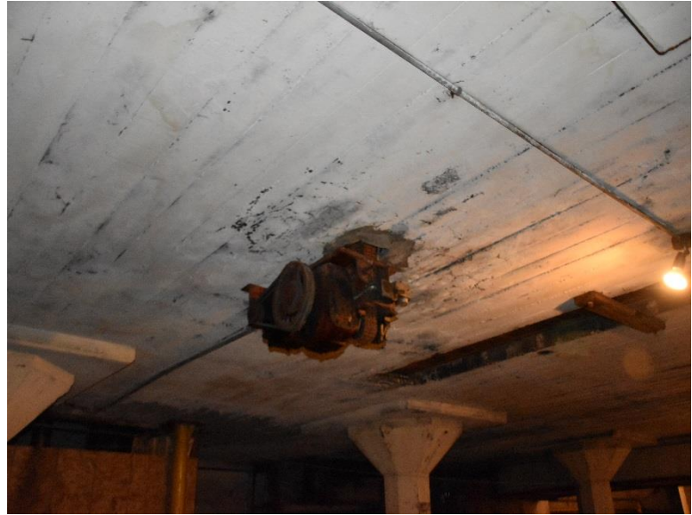
Representative Remnant Chain Hoist and/or Fruit Box Conveyor System in Warehouse
