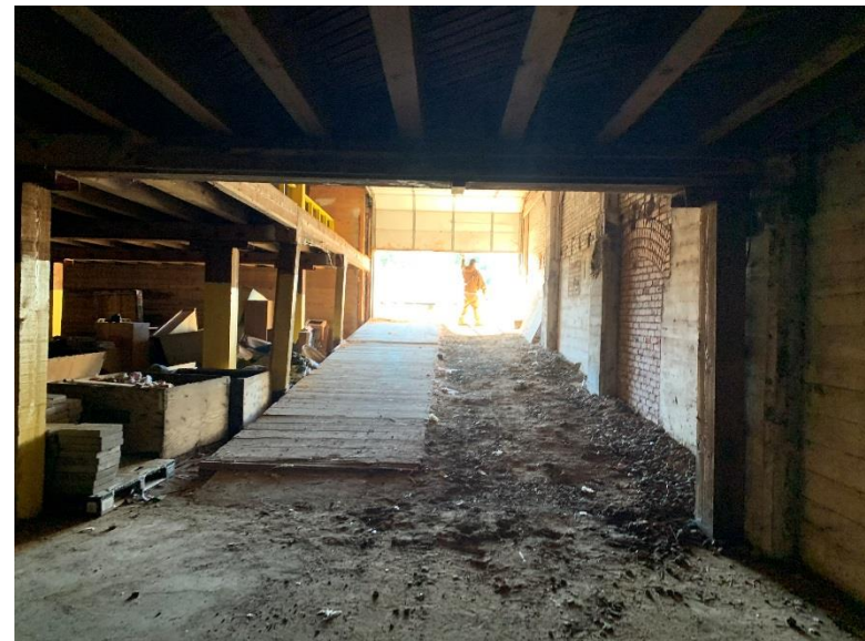
Loading Ramp in Southern Portion of Warehouse Basement – View to West
