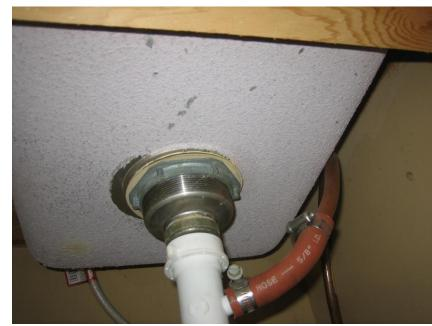
Photo 2: ACM Sink Undercoating in the Breakroom.
