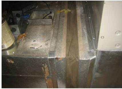
Photo 7: View of the non-ACM vibration dampener in attic.
