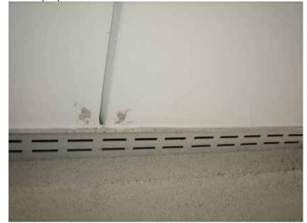
**Photo 12:** View of the drive-thru ceiling with non-ACM drywall / joint compound (HA 17).
