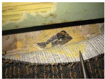
**Photo 10**: Non-ACM floor tile under carpet with ACM black mastic (HA 14) in the safety deposit vault.
