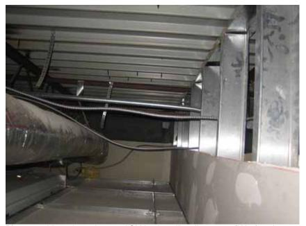
**Photo 4:** View above the non-ACM lay-in ceiling tile system (HA 3) and non-ACM drywall joint compound (HA 4).
