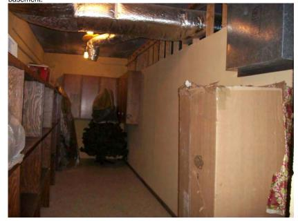
**Photo 8:** View of the non-ACM drywall/joint compound (HA10) located in the basement.
