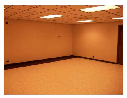
**Photo 6:** View of the non-ACM 2'x2' ceiling tiles (various styles HA 5-7) located in the basement.
