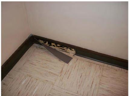
**Photo 3:** View of the non-ACM 12"x12" floor tile with associated ACM black mastic (HA 1) and non-ACM cove base mastic (HA 2).
