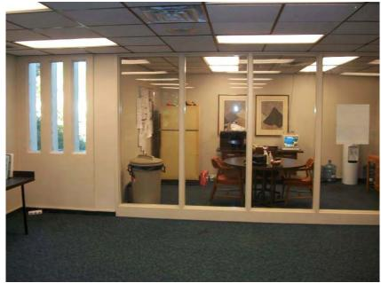
**Photo 9:** View of the non-ACM 2'x2' ceiling tiles (HA 6, 7 and 13), ACM carpet mastic (HA 9), and textured window paint (HA 11) located in the work area.
