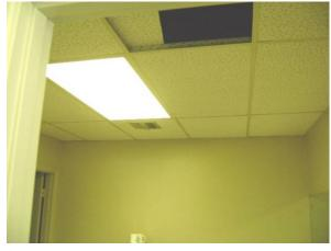
Photo #6 Lighting in 2'x4' drop ceiling tile (white, pinhole, fissure) – HA 03
