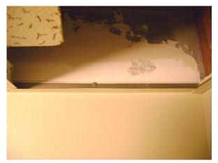
Photo #3 Gypsum Wallboard and Joint Compound ACM (white) – HA 02 and Wall Texture ACM (white) on concrete block – HA 07
