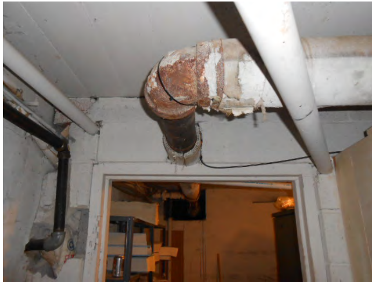
TSI leading out of elevator room to hallway.
