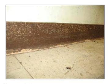
**Photograph No. 8**View of tan 9" x 9" floor tile (and associated mastic beneath), as well as brown cove base
