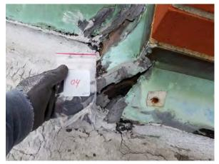
**Photo #3** Sample 04, silver paint and flashing, south canopy.
