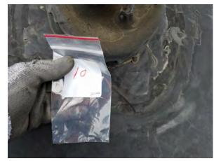
**Photo #7** Sample 10, roof caulk around condenser penetrations, main roof.
