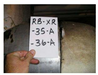
Photo #27 RB-XR-35A and RB-XR-36A – Pipe insulation and wrap are ACM (15% and 4.9% Chrysotile)
