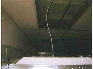
Photo #7 Multiple ceiling systems; 2' x 4' Ceiling tile (white, pinholes, and fissures) and tin ceiling tile above metal lay-in ceiling tile system.
