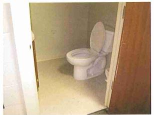
Photo #19 12" x 12" Floor tile (beige w/brown specks) with mastic (yellow) on resilient sheet flooring.
