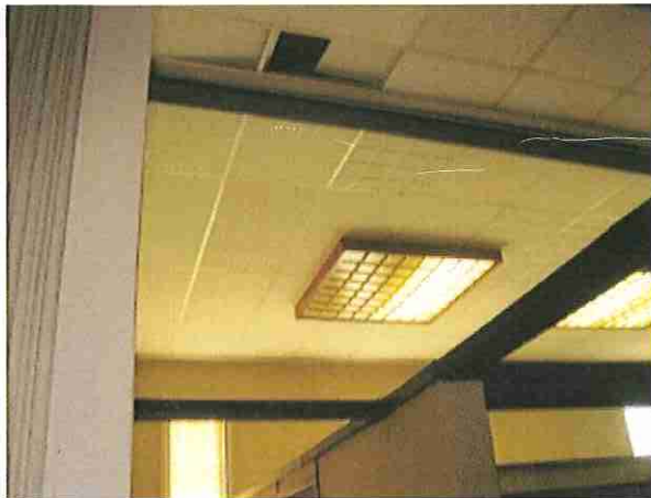
Photo #13 2' x 4' Ceiling tile (white, pinholes, and fissures) and 2' x 2' Ceiling tile (white, pinholes indents, small squares).
