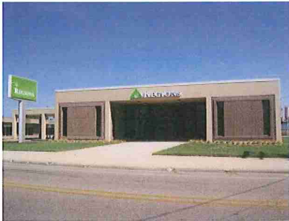
Photo #1 Front of bank.
