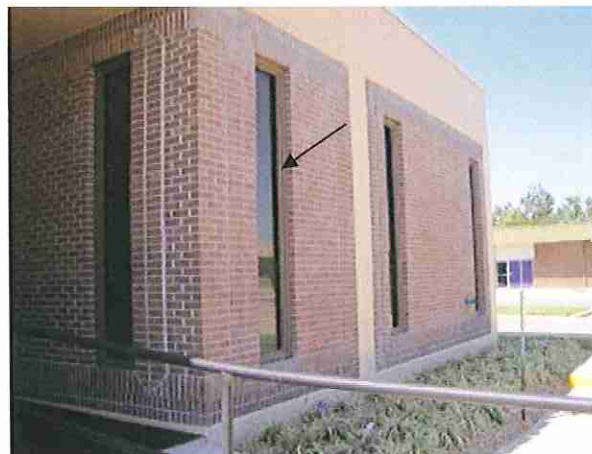
Photo #17 Exterior window caulk (black) and exterior building caulk (gray).
