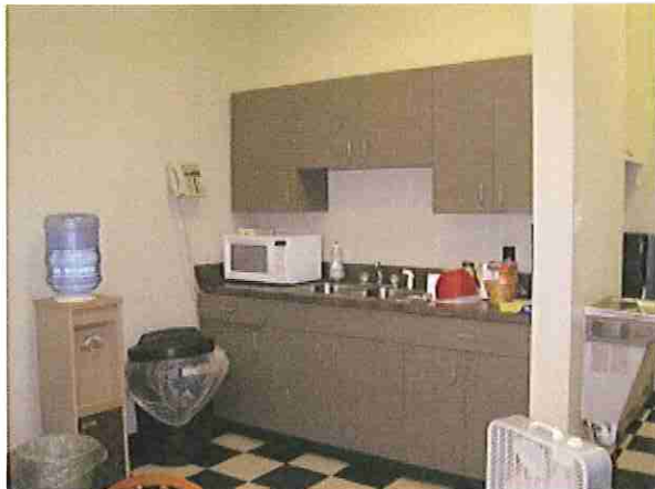
Photo #9 Sink undercoat (white) and 12" x 12" floor tile (black/white checker) with mastic (black).
