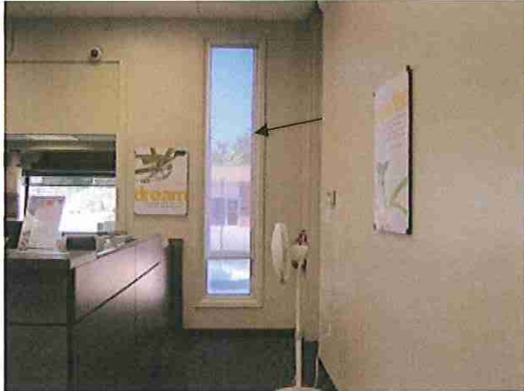
Photo #7 Interior window caulk (black).
