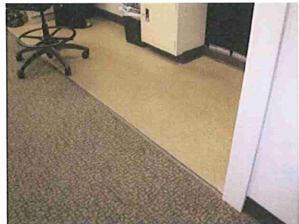
Photo #6 Resilient sheet flooring (brown) and cove base mastic (tan).
