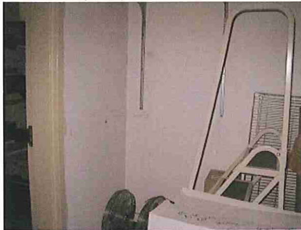
Photo #15 Texture associated with concrete (off-white, semi-smooth).
