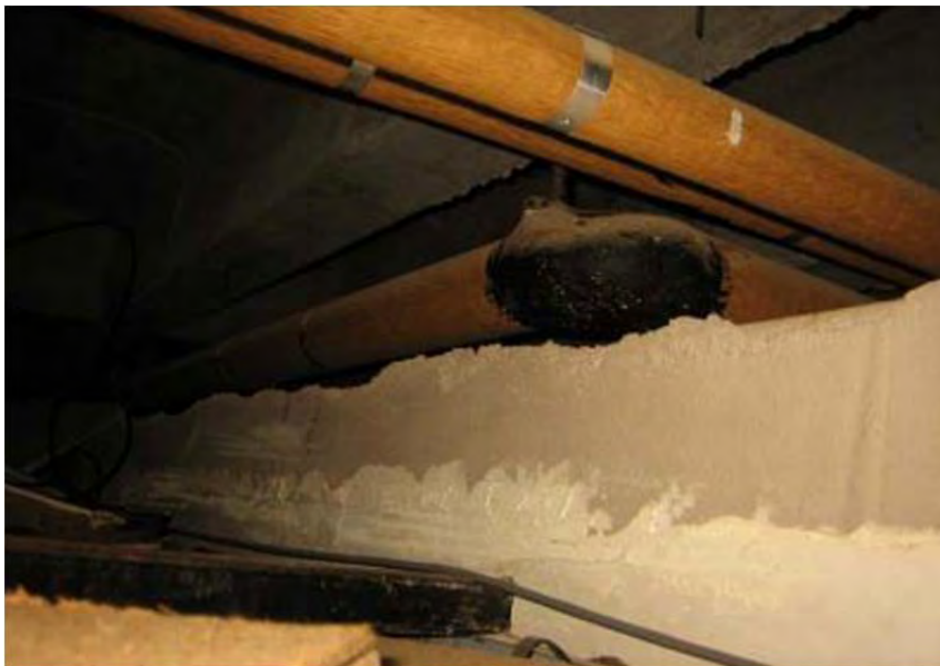
Photo 11: Non-ACM plaster wall in 2 nd floor.
