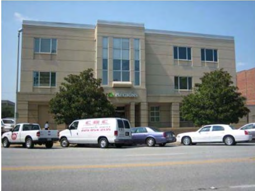
Photo 1: Albany Main RFC 003901.
