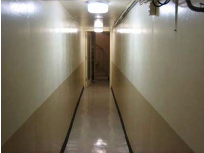
Photo 9: Drive-through teller tunnel, 2 nd layer flooring is ACM.
