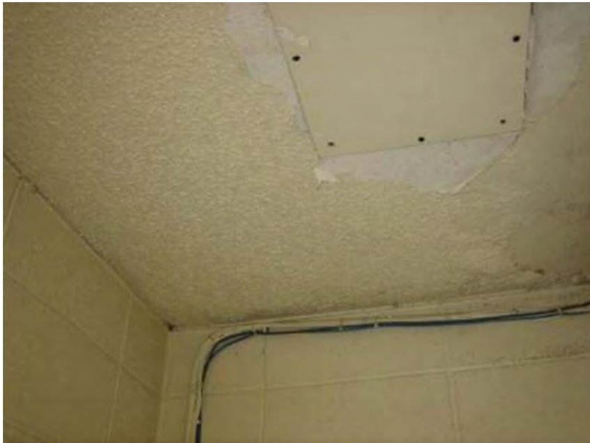
Photo 7: Non-ACM ceiling texture in drive-through teller booths.
