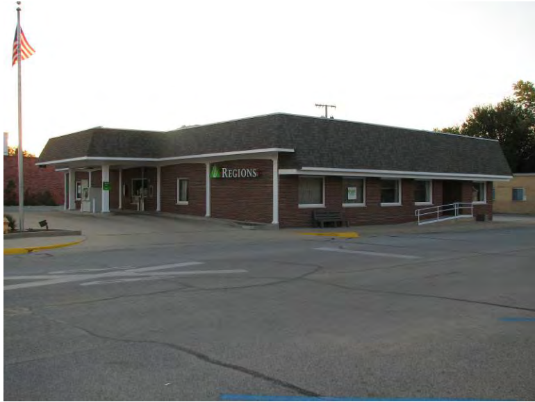
Photo 1: Exterior of the Regions Bank branch. Asbestos-containing joint compound is present on painted drywall seams throughout the structure (not observed on wallpaper seams).
