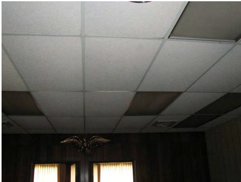
Photo 3: An example view of 2' x 4' drop ceiling tiles in the building.
