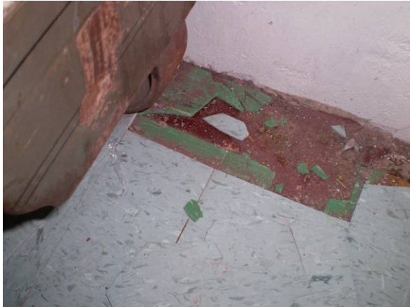
Photo #13 ACM 9"x9" Vinyl Floor Tile, Forest Green (HA#3)
