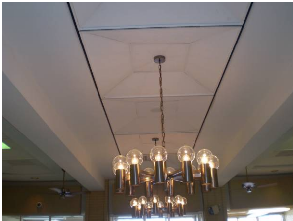
Photo #29 Lobby Ceiling
