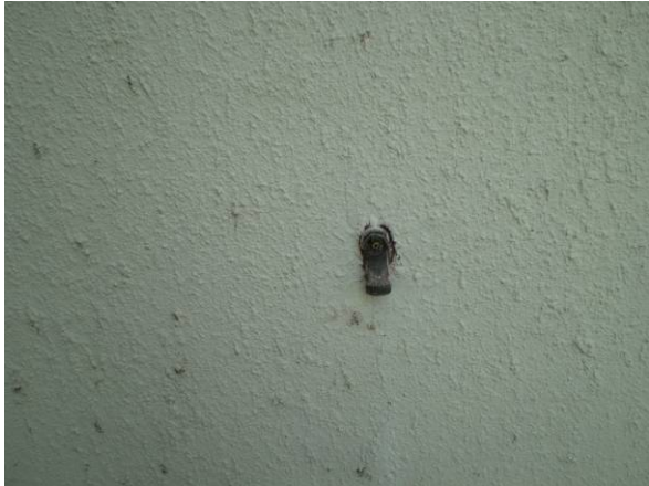
Photo #19 Stucco on rear Exterior Wall (HA#15)
