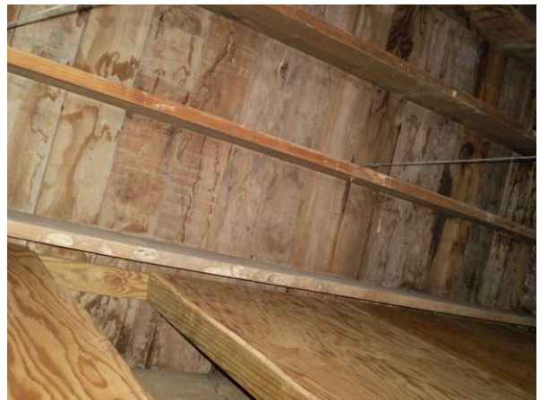
Photo #42 Attic Ceiling
