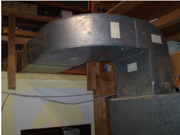
Photo #37 HVAC Ducts in Attic
