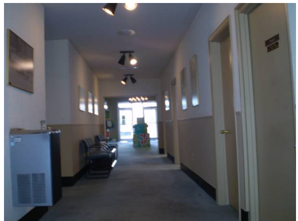
Photo #6 Hallway, Showing Textured Wall, Cream (HA#17) & Cove Base, Brown (HA#19)
