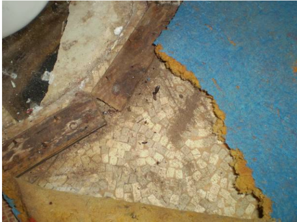
Photo #15 ACM Vinyl Floor Tile Cream & ACM Linoleum, Gold/Beige (HA#13 & 14)
