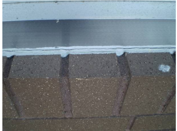
Photo #16 ACM Window Caulk, Gray, Front of Bank (HA#11)
