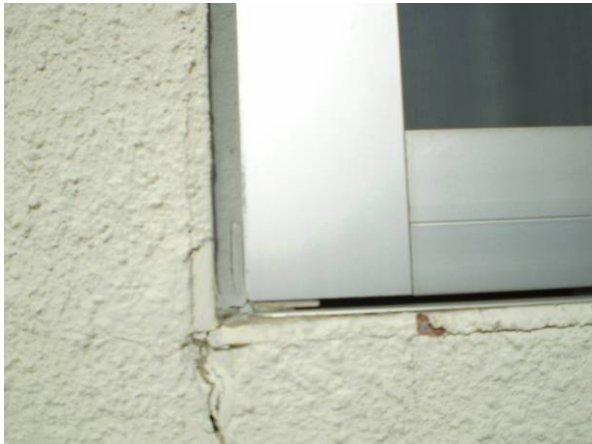
Photo #45 ACM Window Caulk, Light Gray (HA#12)
