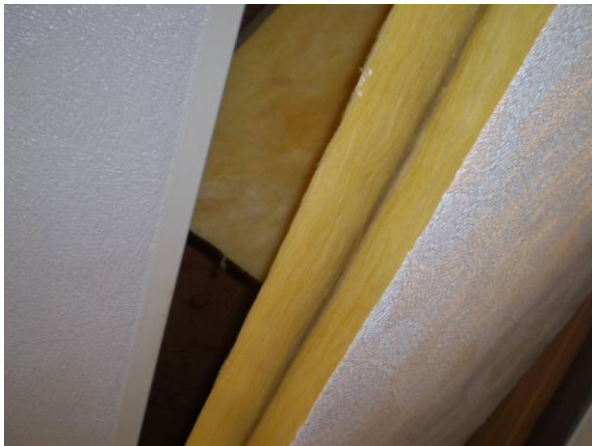
Photo #27 Fiberglass Panels in Office 3
