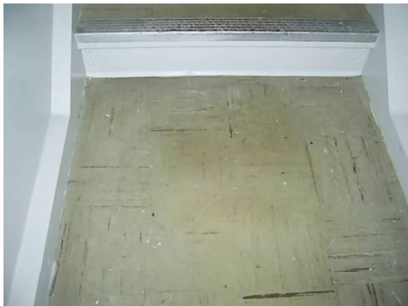
Photo #5 9" x 9" floor tile, tan/brown located in the front stairwell.
