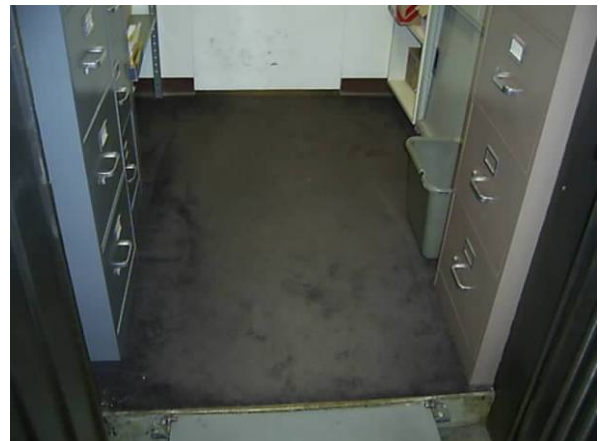
Photo #6 Carpet mastic (black/brown) located in the teller vault.
