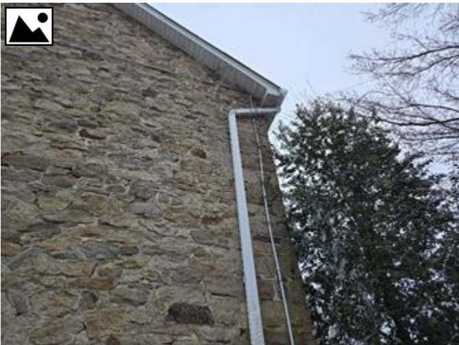
Water Control - Gutter/Downspout
