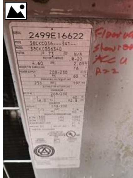
HVAC - Heating System 2 Data Tag
